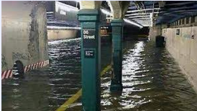
Subway station in New York is shown flooded with water during Hurricane Sandy. 2012/10/29
