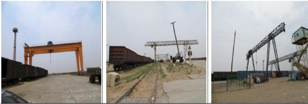
Figure 2.3 Cranes at Terminal 1
