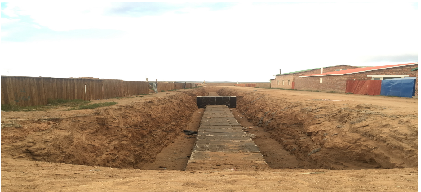
Figure 8: New sewerage system
