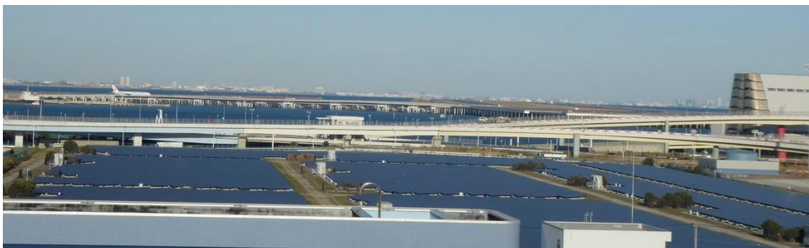
Figure 20. Ukishima Solar Power Plant.
